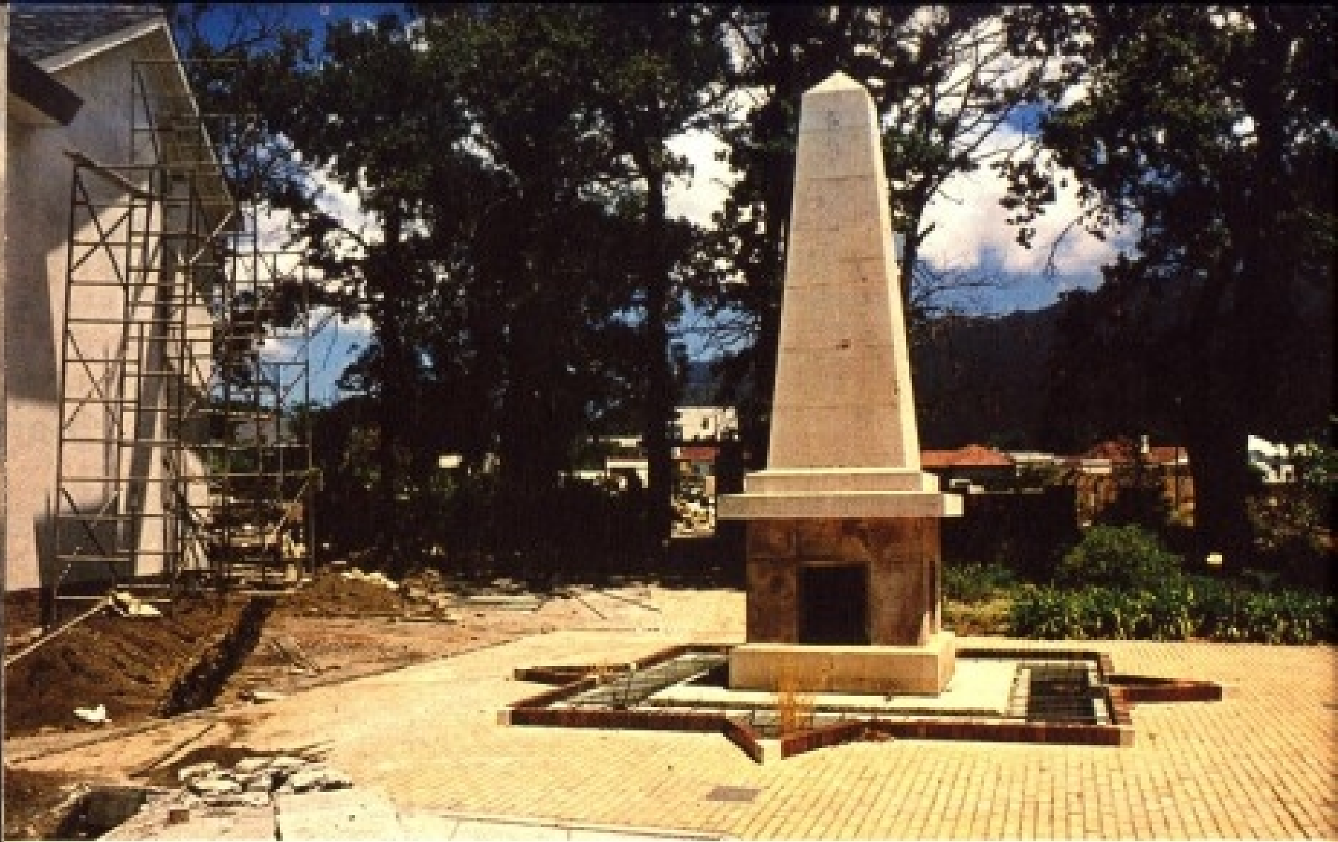
The Herschel Monument during building operations at the Grove Primary School, Claremont. - Dr Patrick Moore
