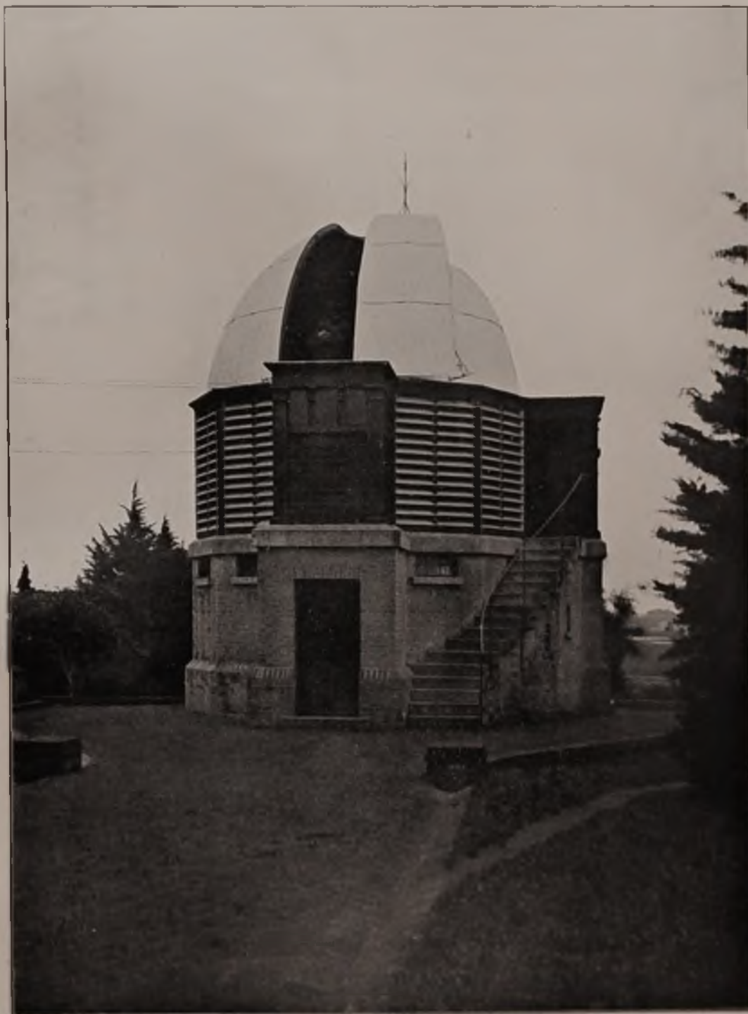
THE HELICONIA OBSERVATORY. General View from the South-east.
