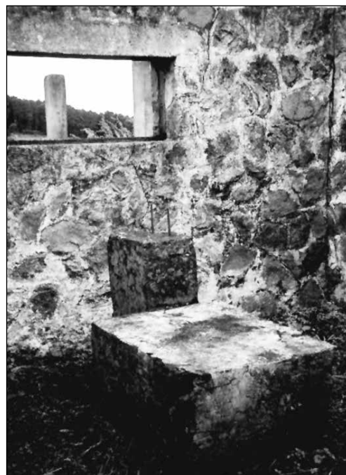
The sturdy stone structure still houses the pillar with screws on which his telescope had been mounted.
