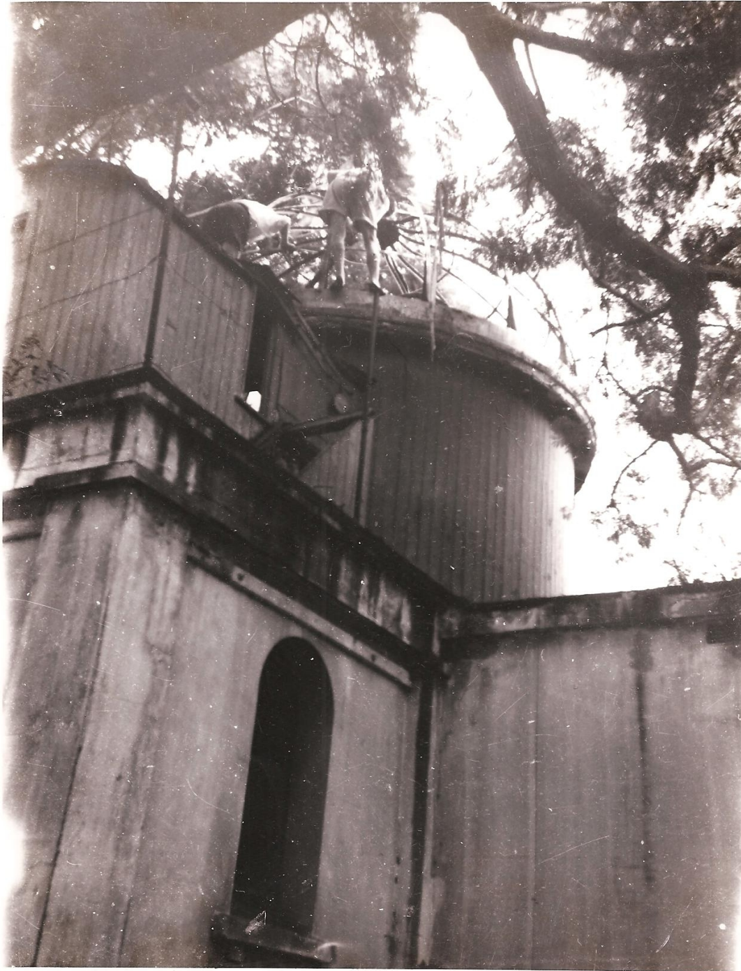
Probably the very last photograph ever taken of the old Observatory building just prior to demolition. The dome is being stripped by members of the local Astronomical Society. Taken with a box camera, the negative has been rediscovered and presented to the Local History Museum Durban. Taken by Mr G Roberts in mid-1957. (by permission of Local History Museum)
