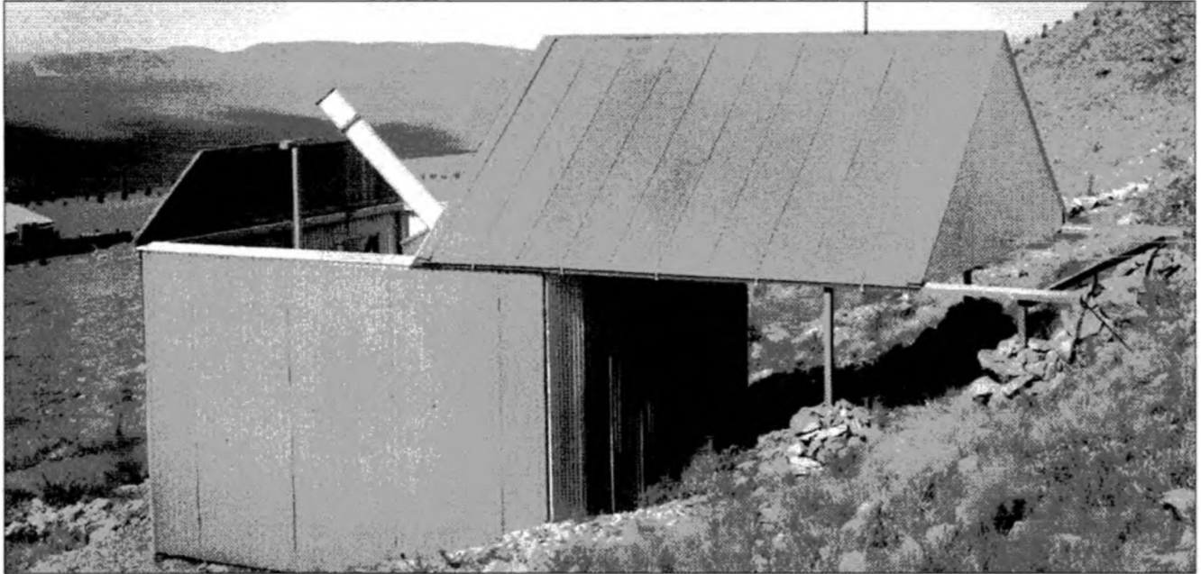
Fig. 31: The 9-inch Grubb telescope in its wood and iron housing with sliding roof. This instrument was known as the Reunert telescope (CSIR Archives)
