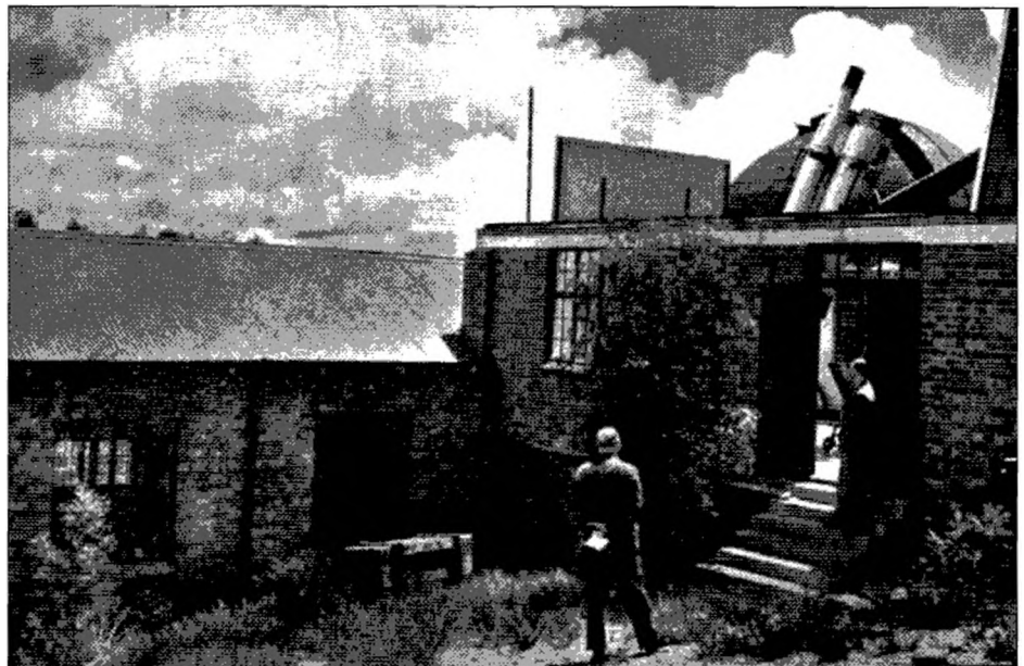
Fig. 50: The Rockefeller double astrograph having two 16-inch photographic reflectors with focal lengths of 90 inches (ref 46)
