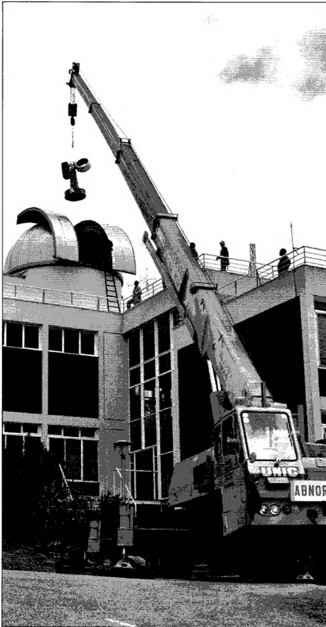
Fig. 111: Removing the Boller and Chivens telescope for re-installation at the SAAO Observatory in Sutherland (Greg Roberts)
