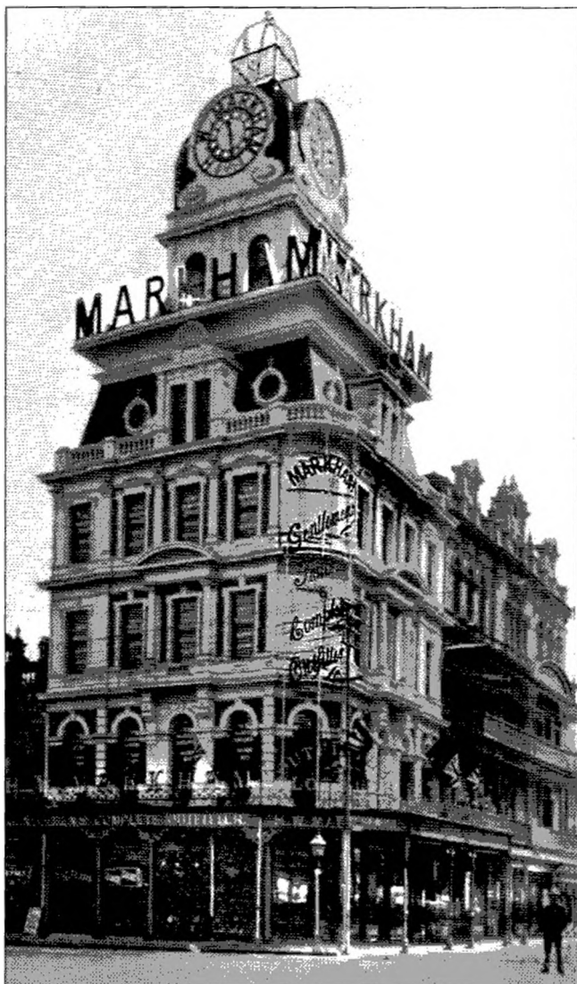
Fig. 101: At the beginning of the 20th Century many Johannesburgers, including the staff of the Meteorological Station, depended on the prominent clock in the tower of Markham's Building (built on the corner of Eloff and Pritchard Streets in 1895) for correct time
