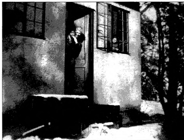
Fig. 77: Mrs Corrie van den Bos at the door of the prefabricated house they erected at the Johannesburg Observatory (block 3 in fig 137) (E Lockwood)
