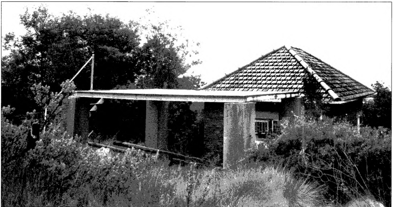
Fig. 123: The platform built to support the two 7,3 m diameter micro-wave parabolic reflectors for the NITR rainfall research project. The building now covered with a tiled roof was erected in 1912 to house the Franklin-Adams 6/7-inch telescope - the concrete pillars supported the sliding roof (author)
