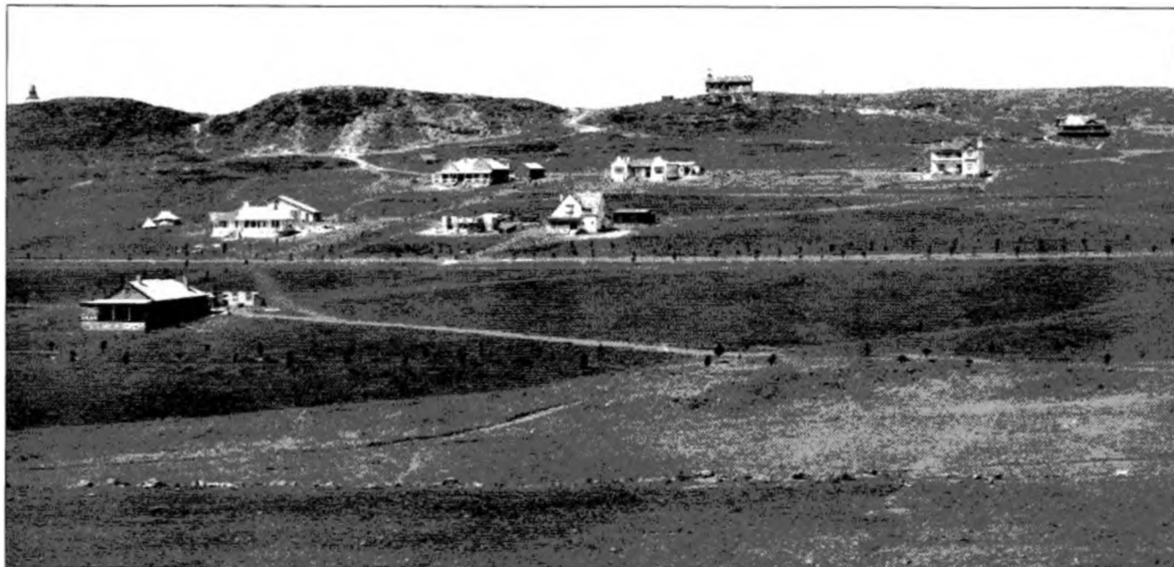
Fig. 25: The two buildings of the Transvaal Meteorological Department at the top of the ridge are accompanied by some of the earliest residences in the new suburb of Observatory (ca 1908) (HE Wood)
