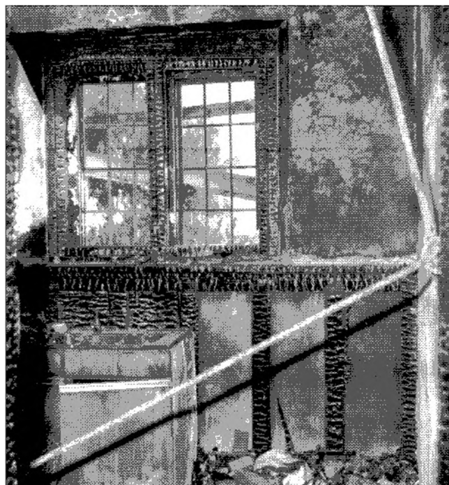
Fig. 132: Fire damage to one of the small rooms in the Baker Library
