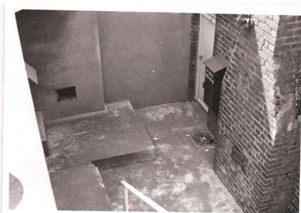
The rear doors of the two Assaying ovens - all that is left of the original furnaces. Photograph by Author
