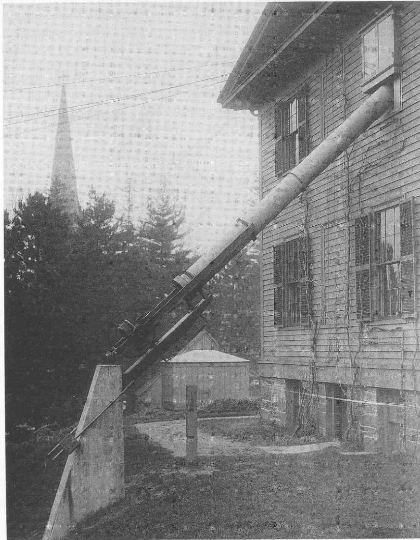
Figure 7.26. Gerrish student telescope mounted in the side of a classroom building. Photo from Harvard College Observatory.
